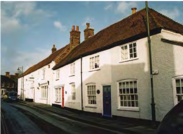
Listed buildings along the north side of The Square, facing west
