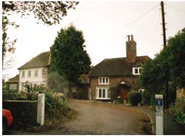
Entrance to Old Rectory Close
