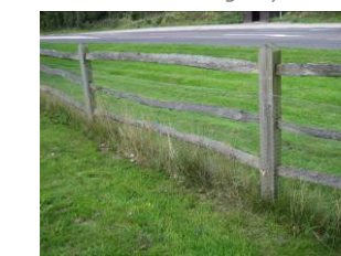
Hardwood post and rail fencing
