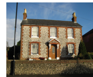
Flint cottage with slate roof
