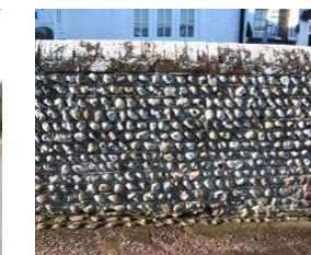
Flint wall with half round brick coping
