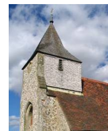
Shingles on church roof
