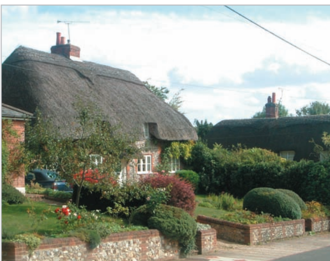
A sequence of linear and nucleated settlements are located above the floodplain, with housing constructed from traditional brick, flint and thatch materials.
