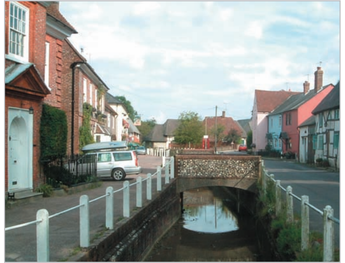
Frequent river crossing points on historic bridges.
