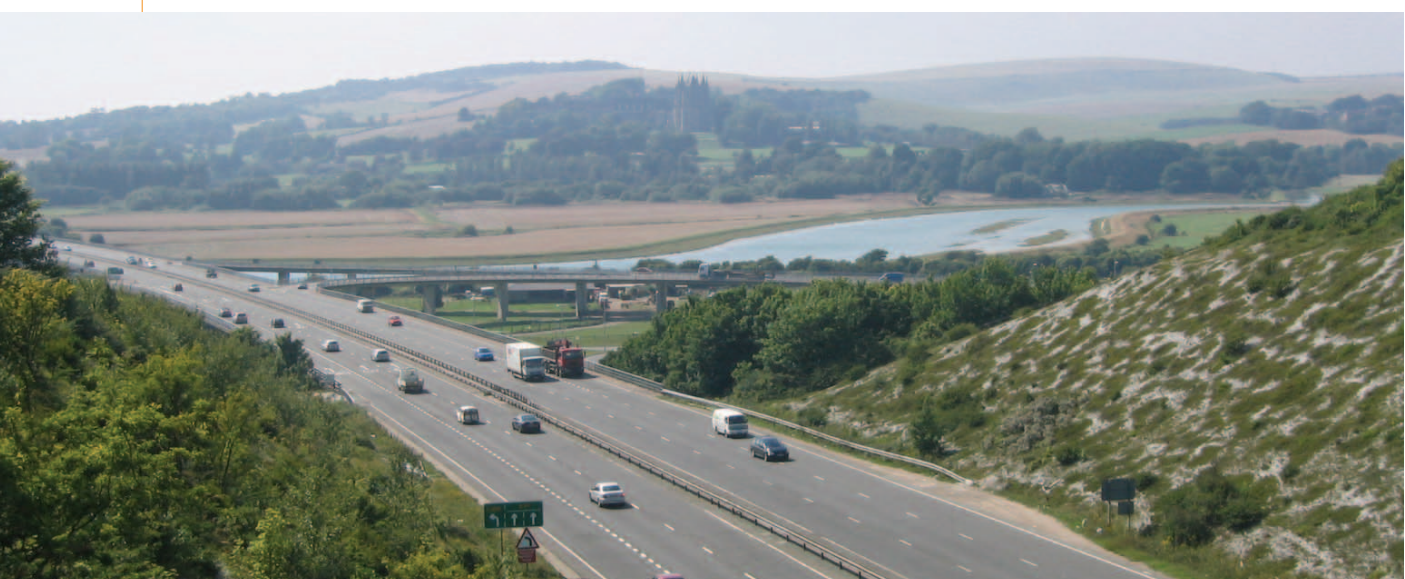
The A27 Trunk Road crossing of the River Adur near Lancing College, Shoreham-by-Sea
