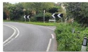
Junction from bridge (no traffic visibility)
