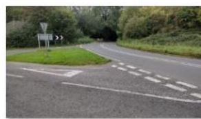
Bend sign is small and close to bridge
