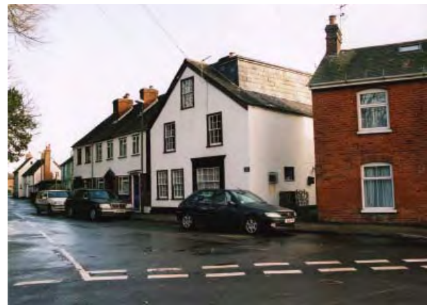
Over-sized “dormer” at No. 1a River Street
