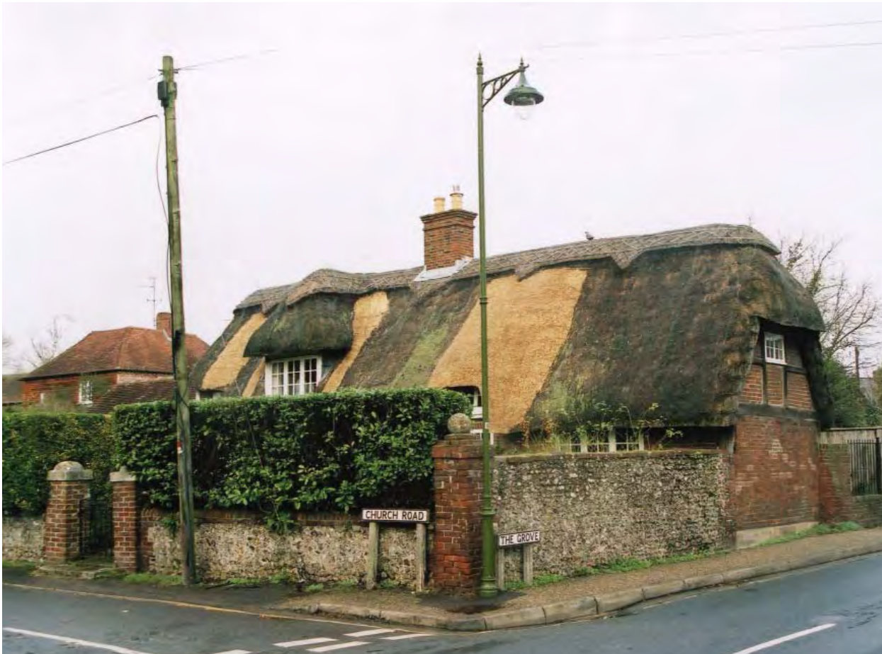
Overhead cables in Church Road
