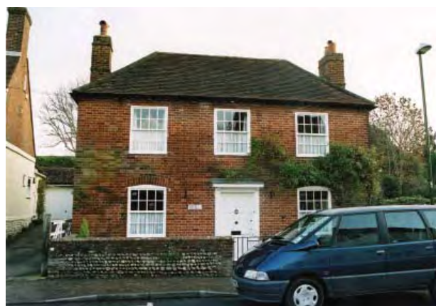
Churchers Farm House, North Street
