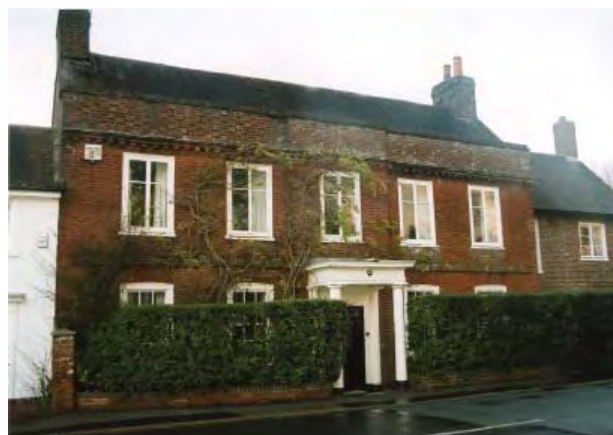
Mile End House, Foxbury Lane
