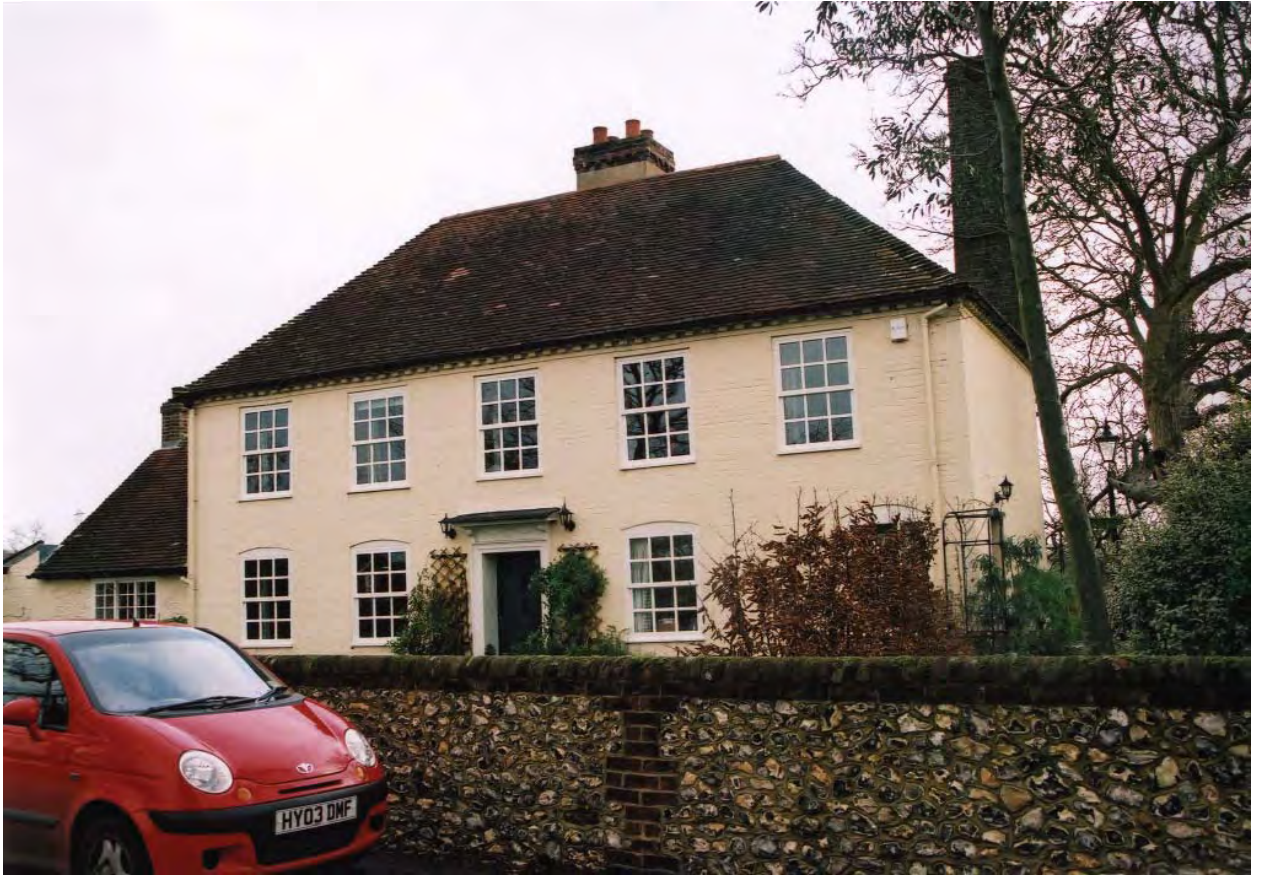
Former engine house lies behind Watersmeet
