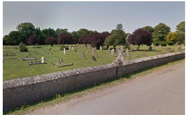
Historic flint and stone walls surround the cemetery, establishing an architectural link to medieval cemetery walls and serving to deter grave robbers.
